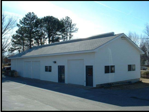
Exterior Renovation, USDA FS, Salem, MO
