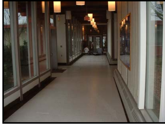
Flooring Renovation USDA FS, Delaware, Ohio
