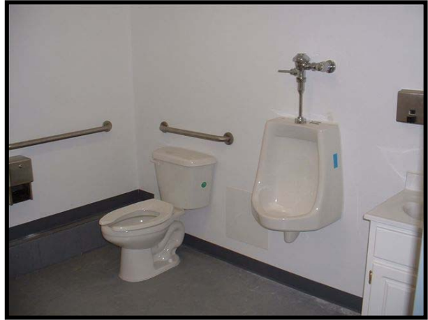
Interior Renovation, USDA FS, Salem, MO
