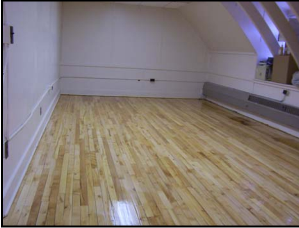
Hardwood Floor Installation, Lansing NOSC, MI
