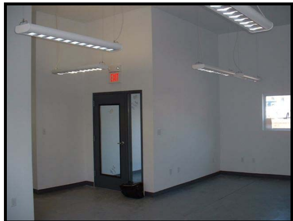
Interior Renovation, USDA FS, Salem, MO
