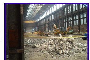
Selective Demolition Allis Chalmers, West Allis, WI
