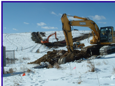
HDPE Header Pipe Installation Delafield Landfill, Delafield, WI
