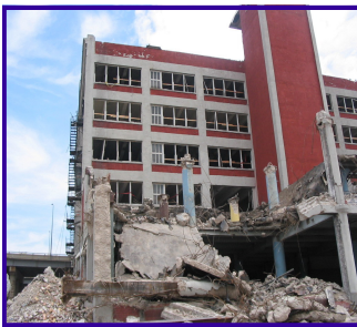
Former Allied Glove Building Demolition, Milwaukee, WI
