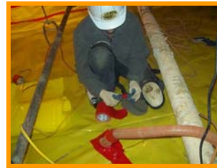
Decontamination Services and Vapor Barrier Installation
