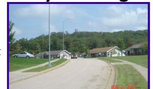
Housing Extension Area Ft. McCoy, WI
