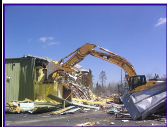
Demolition of the Former ELF Facility Clam Lake, WI
